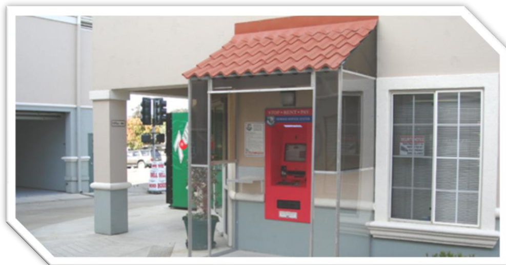
Figure 6: Vestibule Enclosure Installation
